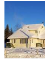
Power for Fort Chip Homes
