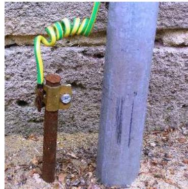
A typical ground rod (left of gray pipe), consisting of conductive steel rod driven into the ground. Below is a ground plate which does the same thing but is easier to install.
