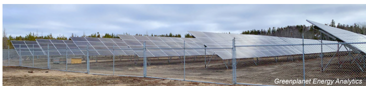
Fort Chipewyan Solar Farm under construction.
