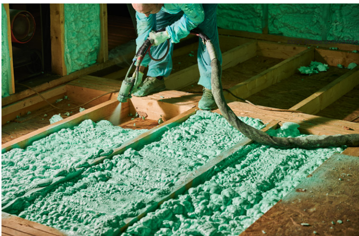
Spray foam insulation
