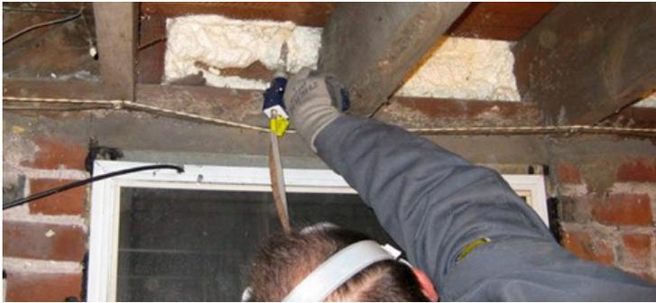
Technician installing spray foam onto a basement header, in between the joists (an area called a rim joist).
